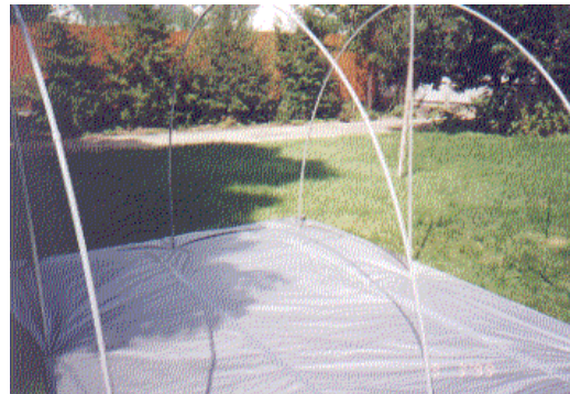
2. Ribs & end posts over stakes.
